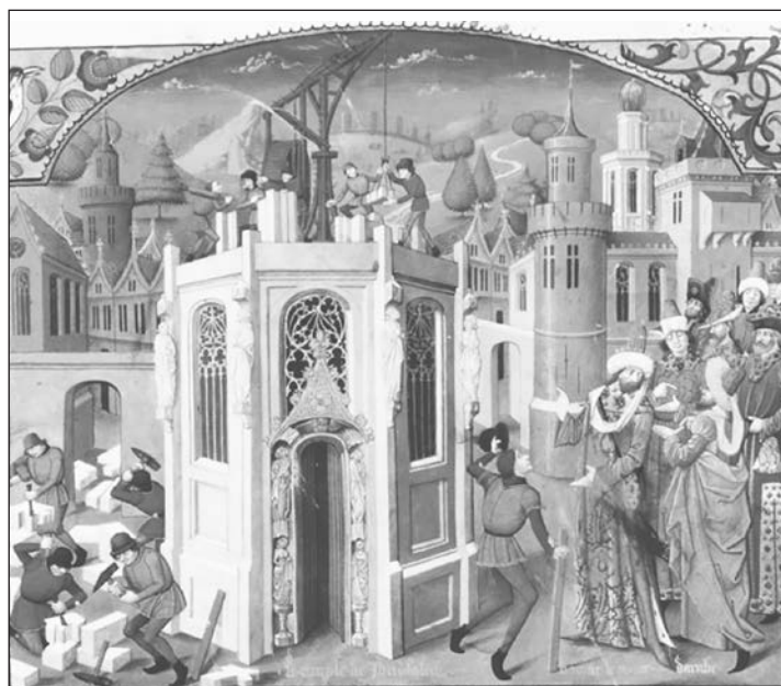
[An illustration showing the construction of a Crusader church in Outremer. It is taken from the chronicle History of Deeds Done Beyond the Sea , produced for Western rulers. It was written by the Archbishop of Tyre, part of the Kingdom of Jerusalem]
